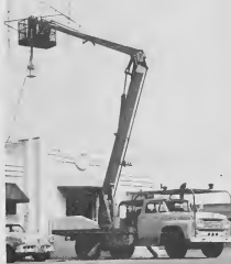
THE VERSATILITY of Lago's "giraffe" was displayed when the Marine Office antenna needed repair. E VERSATILIDAD di e "giraf" a wordo demonstra ora e antenna tabatin mester di mantencion.
